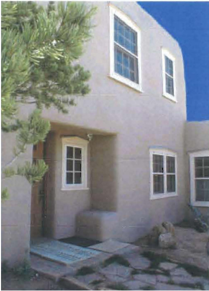
Fig. 17. View of renovated garage into family room and apartment above.
