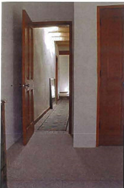
Fig. 13. Hallway seen from the children's room. Note long skylight over vigas, washing the wall in daylight.
