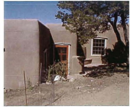
Fig. 16. View toward back of house showing door to new hallway and existing living room window, right.
