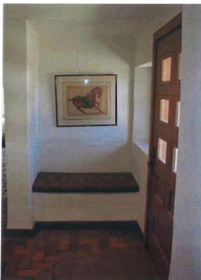
Fig. 19. View of entry to former garage space. The door is extra wide to make up for its low height. The ceiling here is only 7 1/2 ft. high (2.25 m).
